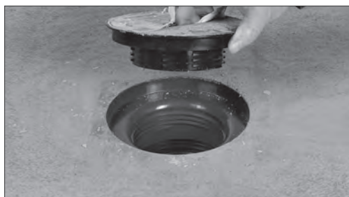
Remove Coring Plug
