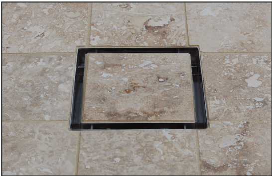
The tile-in drain head installs like a standard drain head, but provides the look of a seamless tile floor.
