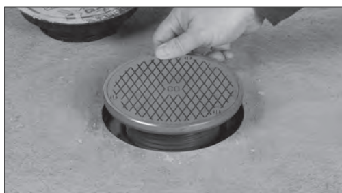
Install Finish Fixture
